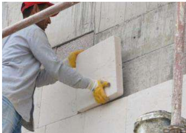
Figure 5. Application phase of perlite lightweight insulation concrete [URL-6]
