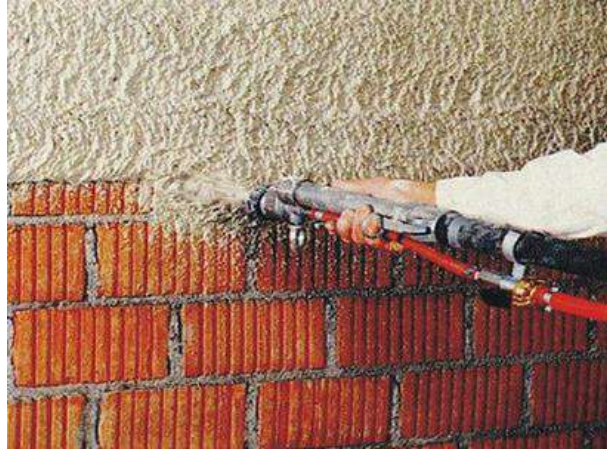
Figure 4. Perlite plaster application phase [URL-5].
